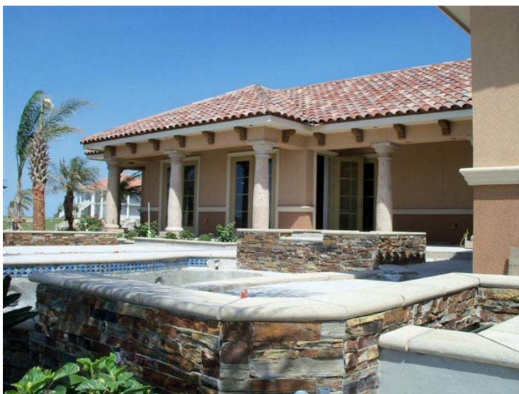
Backyard of Scharck residence, nearing completion
